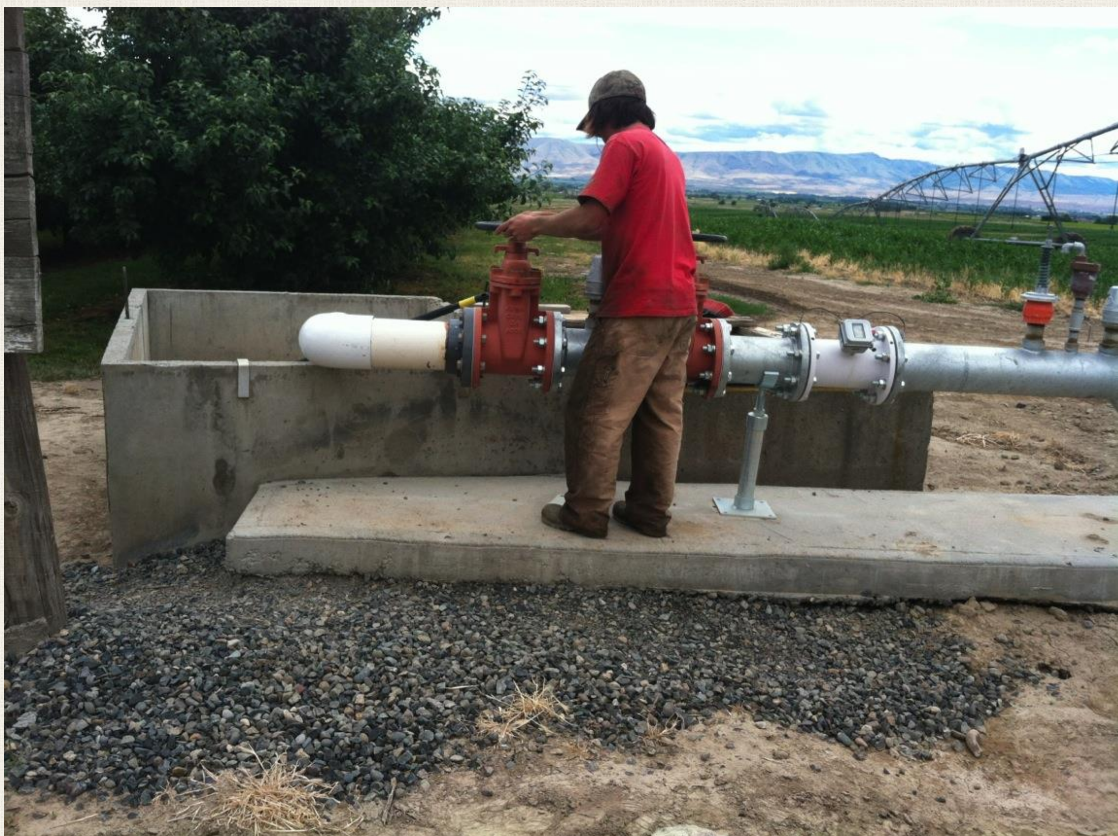
Adjusting the rate of water flow into the water box. This water box filters large debris from incoming water and decreases wear and tear on the pump. The water level must be monitored and adjusted to prevent the pump from drawing air.
