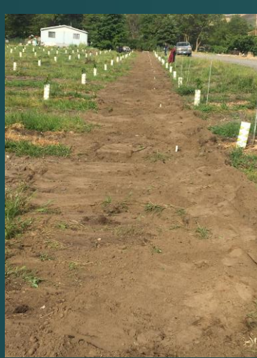
Left: Digging the ditch for the mainline. Middle: Covered mainline with risers sticking up through soil Right: Completed installation
