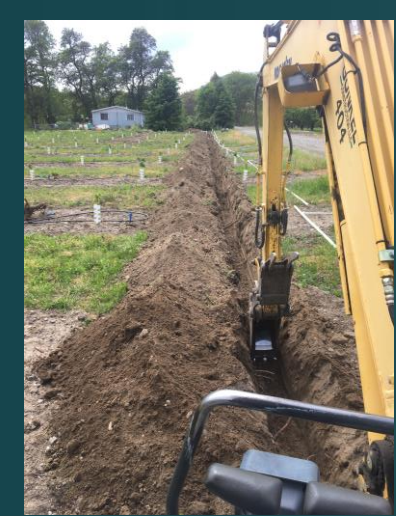
Left: Digging the ditch for the mainline. Middle: Covered mainline with risers sticking up through soil Right: Completed installation
