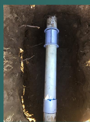
Fixed busted mainline with new coupler
